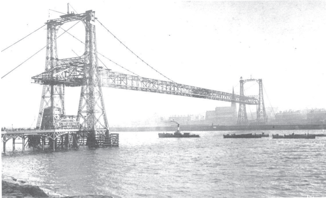
The Transporter Bridge
